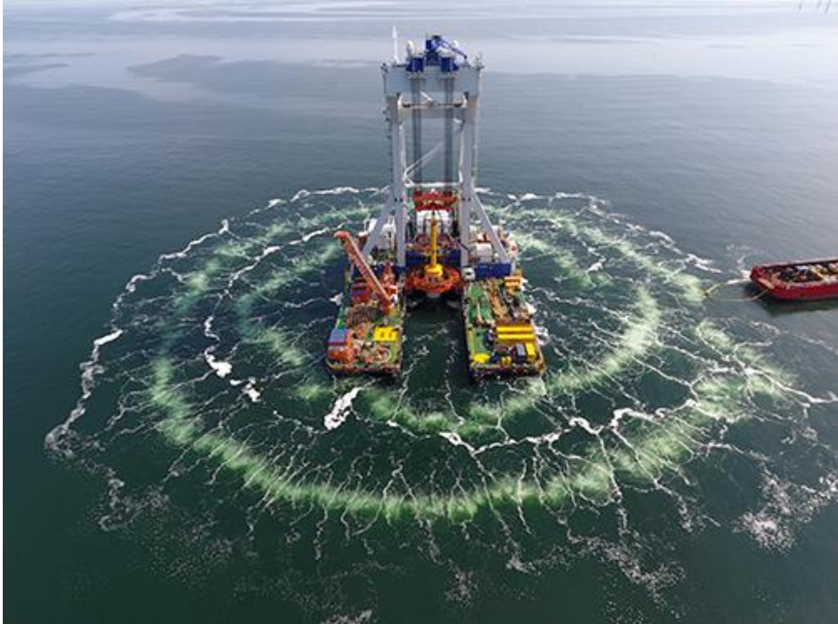
Figur 8-9. Dubbel bubbelgardin (källa: Svanen completes installation works for Danish Kriegers Flak Offshore Wind farm - Ocean Energy Resources (ocean-energyresources.com)).
